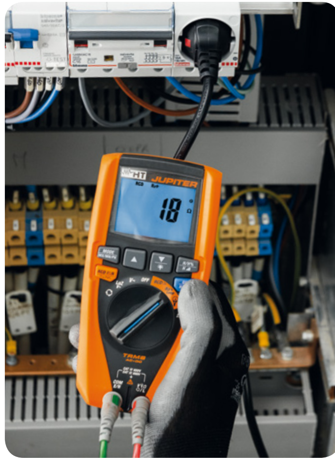
Non-trip earth ground resistance measurement.
