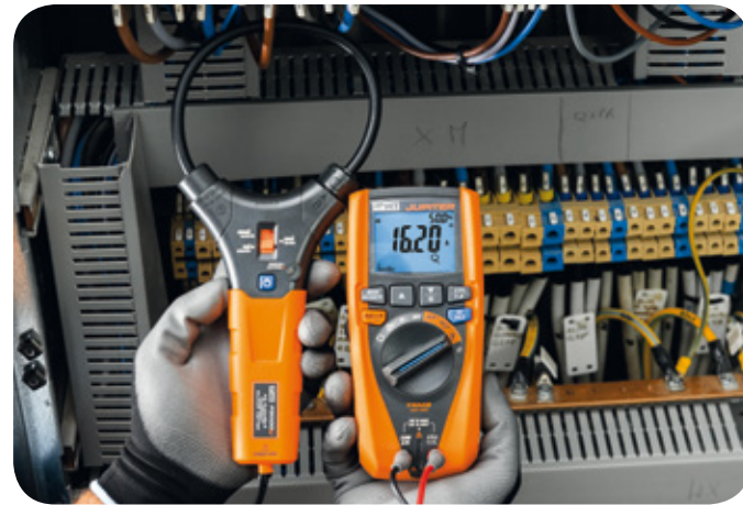
AC current measurement with flexible transducer F3000U.
